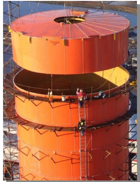
Smooth Wall Bolted Tank being Installed by Eagle Install Crews.
